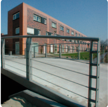
concrete deck without its wearing surface ▼
