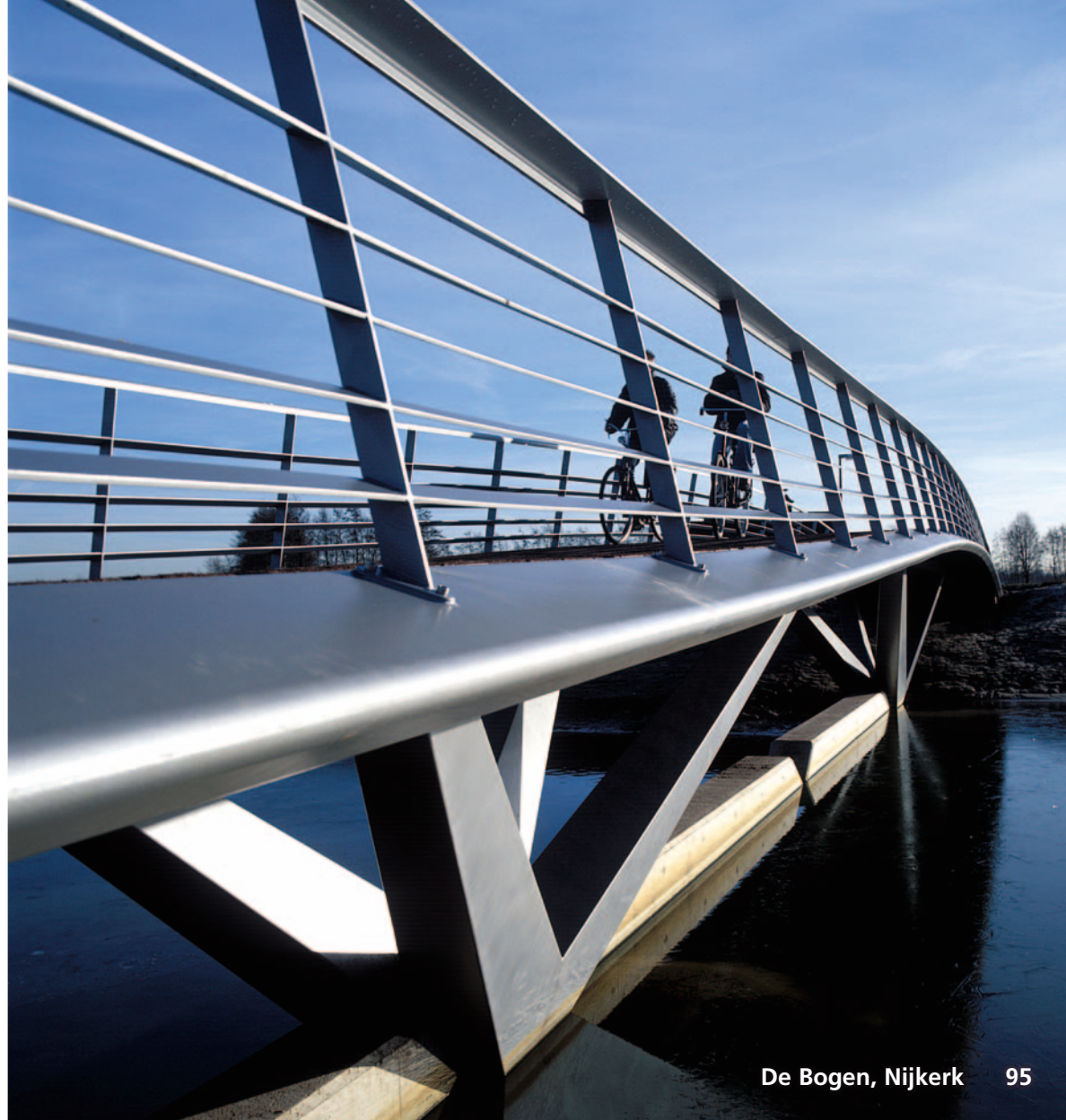
▲ the weir acts as a foundation for the supports inwardly tilted railing ▼
