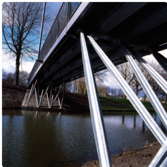
▲ the series of V-shaped supports mounting of the bridge deck ▼
