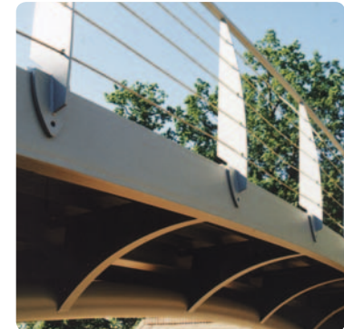
tubular steel beam with cross beams ▼
