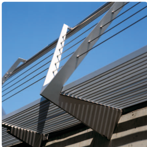
▲ balusters and open steel grid decks
