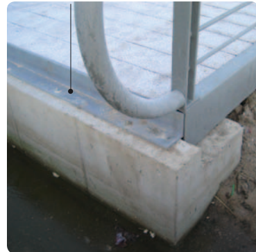
▼ steel angle section, Broekpolder bridge
