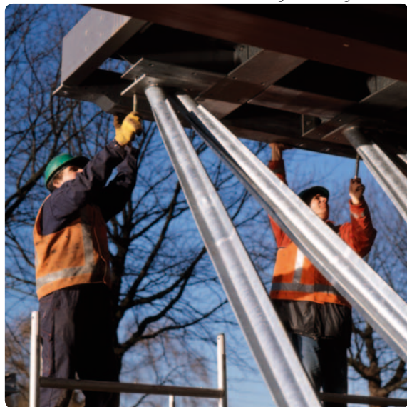
▲ the series of V-shaped supports mounting of the bridge deck ▼
