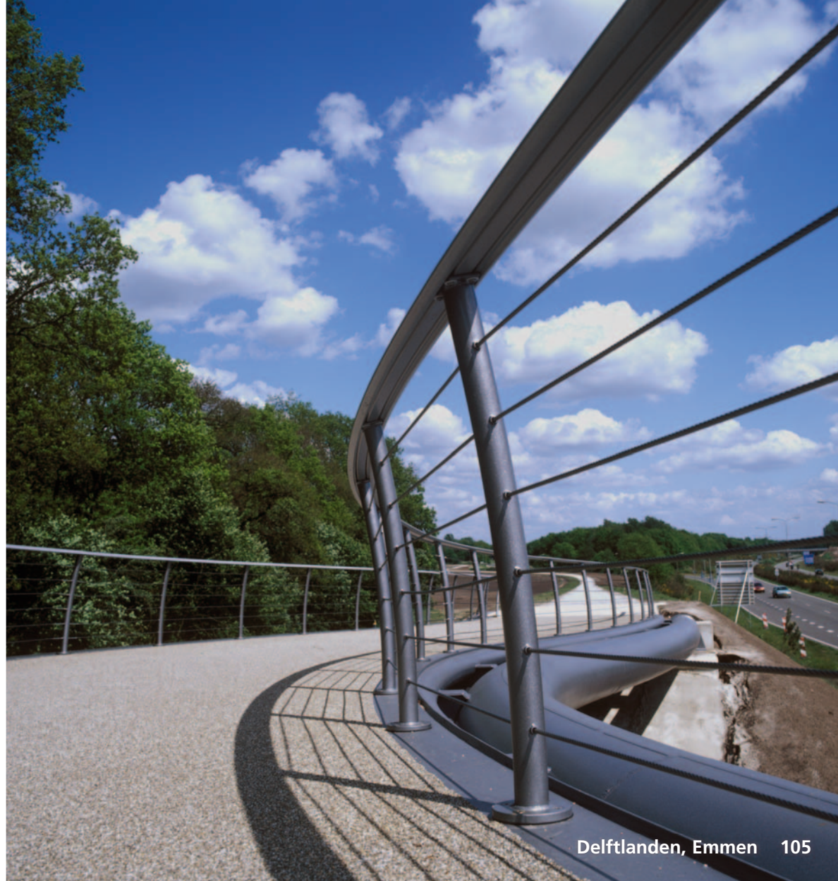
▲ the cables carry the tubular beam cable connection cross section ▼
