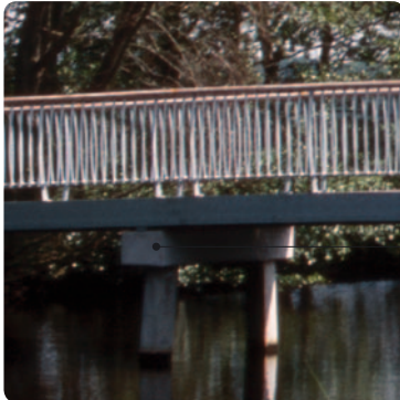
▼ bridge in Meppel, cap on piles bearing
