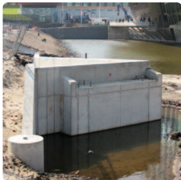
land abutment during construction ▲
