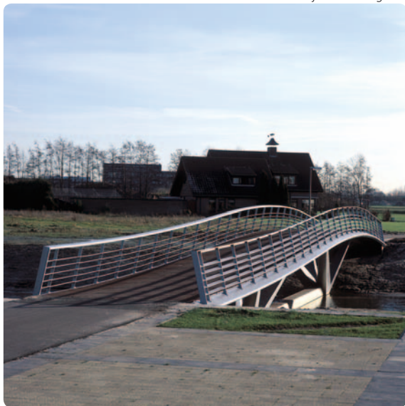
▲ the weir acts as a foundation for the supports inwardly tilted railing ▼
