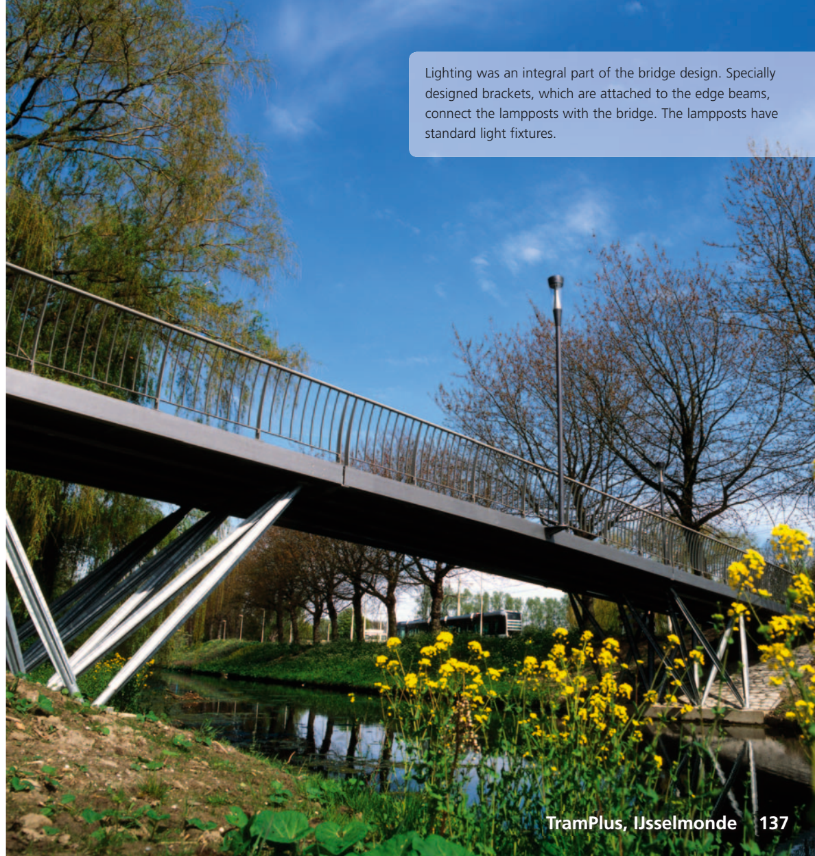
▲ the series of V-shaped supports mounting of the bridge deck ▼
