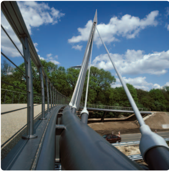
▲ the cables carry the tubular beam cable connection cross section ▼
