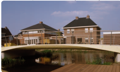
precast self-consolidating concrete edge beam ▼
