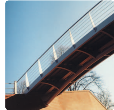
tubular steel beam with cross beams ▼
