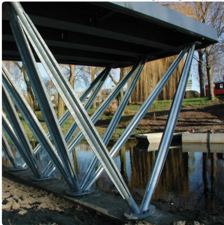
IJsselmonde bridge, mounting of the supports ▼
