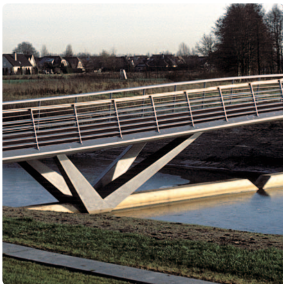
▲ the weir acts as a foundation for the supports inwardly tilted railing ▼
