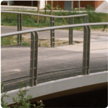
▲ exposed steel edge beams
