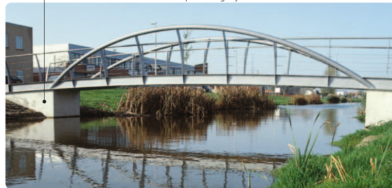
the abutment is placed slightly inwards in relation to the steel beam ▼
